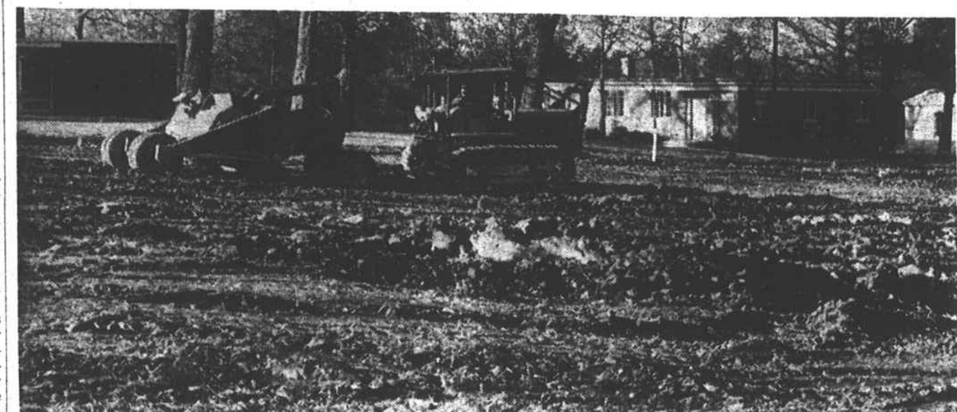
BULLDOZERS AT WORK
