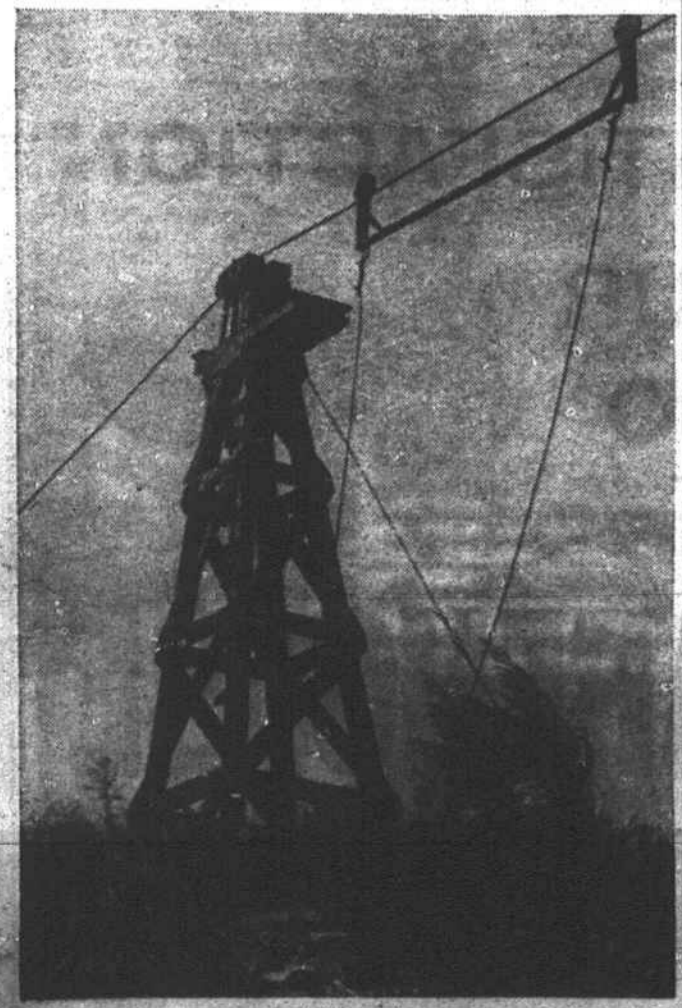
Workers with the Highway Department this week removed the pillar which held one end of the cable stretching across the Roanoke River for generations. (Staff Photos)
