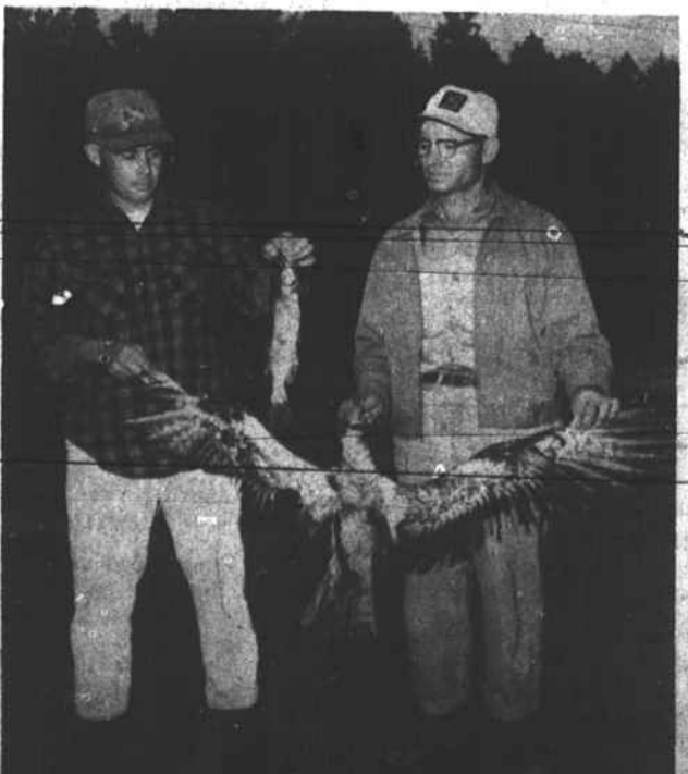
Harold E. Lloyd of Norlina, left, and Raymond E. Eller of Norlina examine the cause of a power failure in Warren County on Sunday. The large bird the two men are holding was electrocuted when the catfish, held by Lloyd, held in the bird's grasp, struck a high-voltage line during a light rainfall. (Staff Photo)
