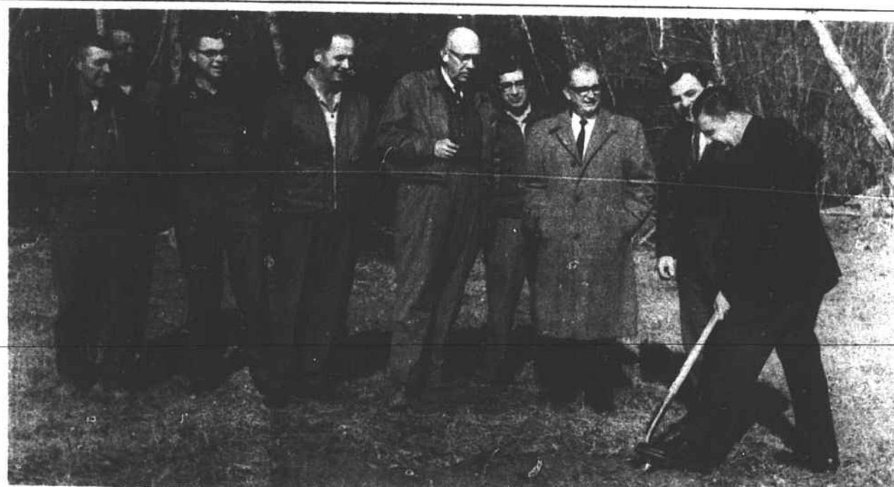
Work was officially started on Warrenton's new sewage disposal plant on Saturday afternoon in groundbreaking ceremonies with Mayor W. A. Miles turning the first shovel of dirt at the site on Horse Branch near its junction with Fishing Creek. Others in the picture are, left to right, D. O. Harmon and Max Taylor, employees of Connell Construction Company; Bill Neal, employee of the Water Department; Hal Connell, contractor; Commissioner Walker P. Burwell, Water Supt. Harold R. Skillman, and Commissioners A. C. Fair and Dixon Ward.
