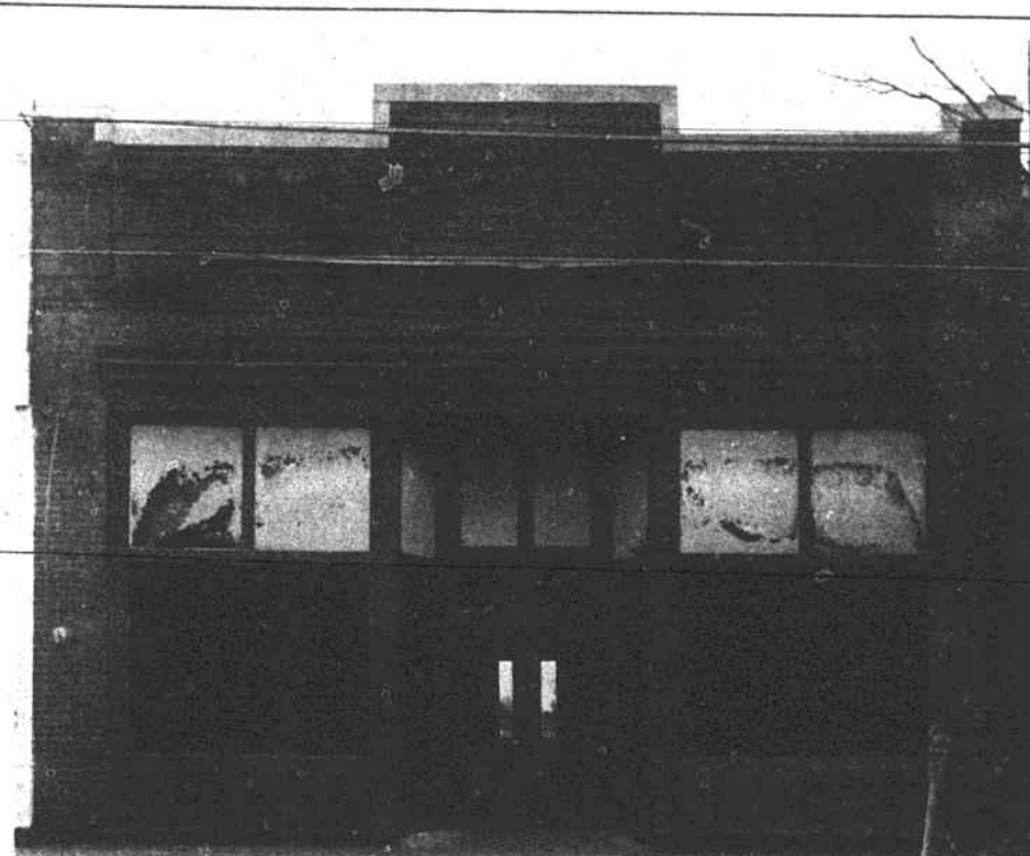
FORMER A&P BUILDING UNDERGOING REMODELLING HERE FOR OFFICES
