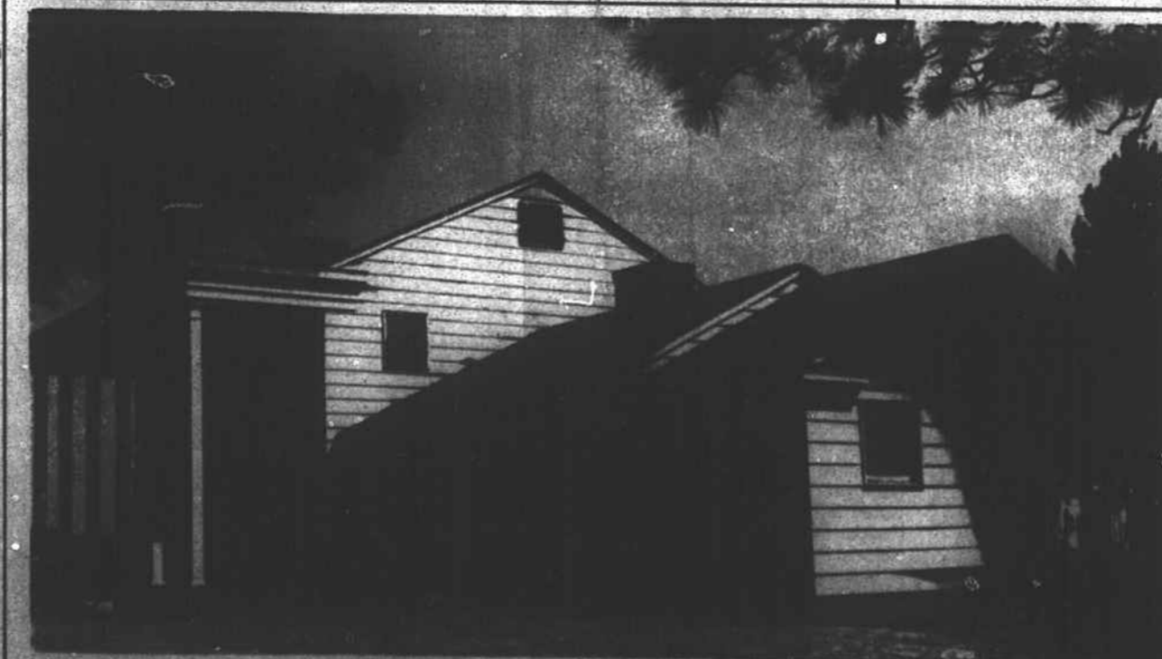
HOUSE SAVED—The home of Carl Aysons of the Liberia Road was saved, with damage only to one wing by the Warrenton Rural Volunteer Firemen who responded to a call around 9 o'clock on Wednesday night.
