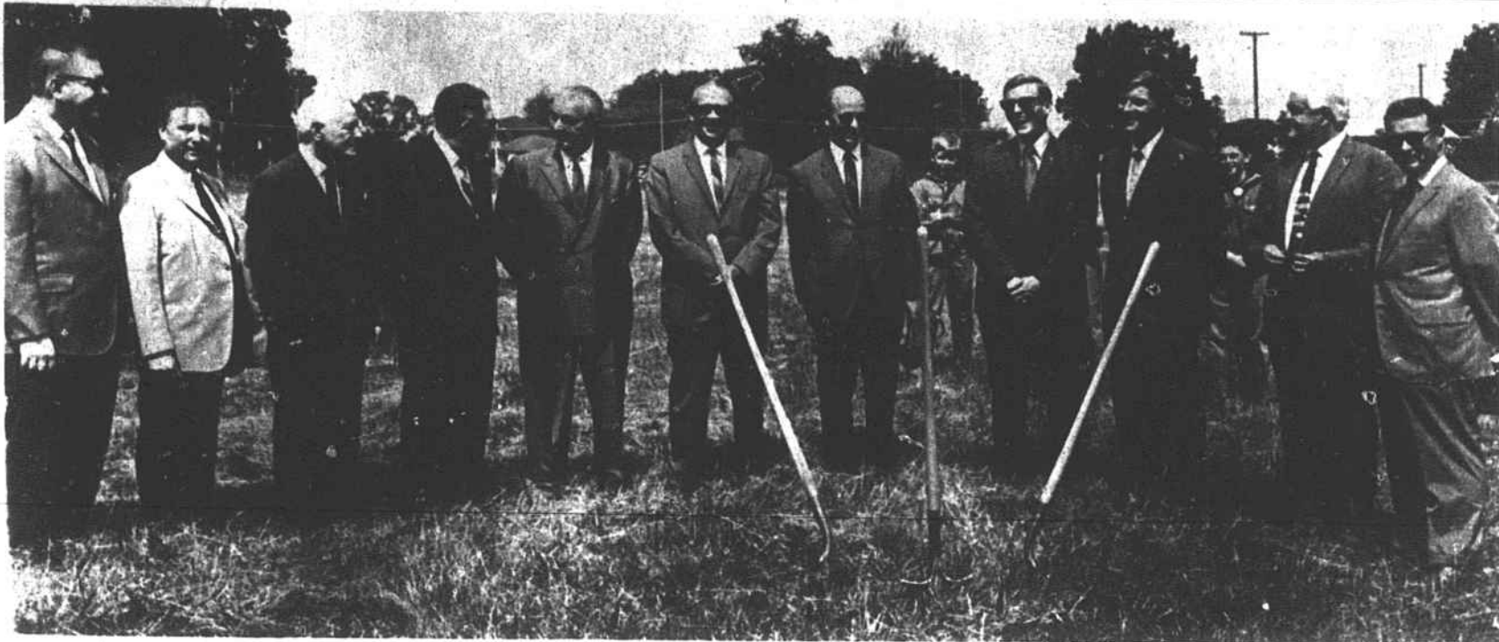
Dignitaries Pictured At Groundbreaking Exercises
