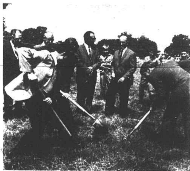
Mayor W. A. Miles, T. E. Cochrane and Jerry Cochrane using their shovels as official groundbreakers for the Cochrane Eastern Plant on the outskirts of Warrenton.
