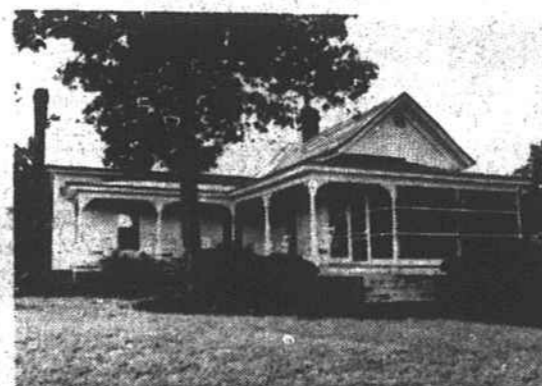
Beulah Vick, Nashville Miss Vick heats her 1854 square foot, 62-year-old home with economical electric baseboard units.
