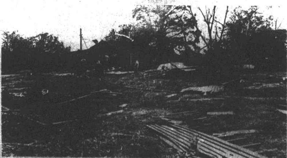
ACROSS THE ROAD, NORTH, WIND SCATTERS DEBRIS
