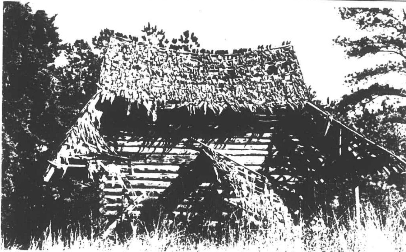
DECAYING CRIB AT NATHANIEL MACON HOME PLACE
