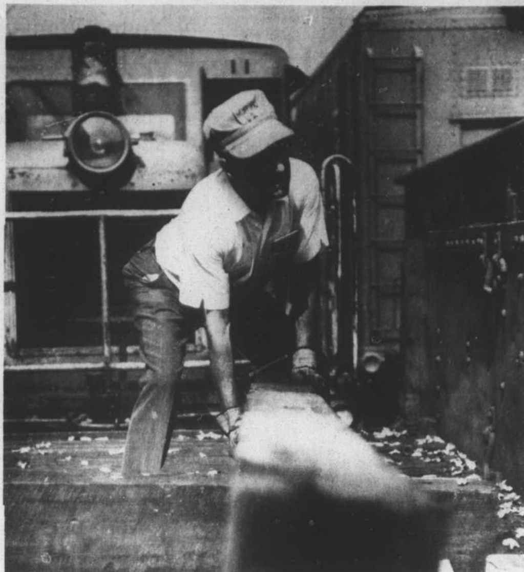
WORKING ON THE RAILROAD — Howard Oakley, driving force behind the Warrenton Railroad, is shown positioning a railroad tie aboard a car hooked to the diesel locomotive which now hauls freight to and from Warren Plains. Hundreds of rail ties have been replaced this year by Oakley and a railroad crew. (Staff Photo)
