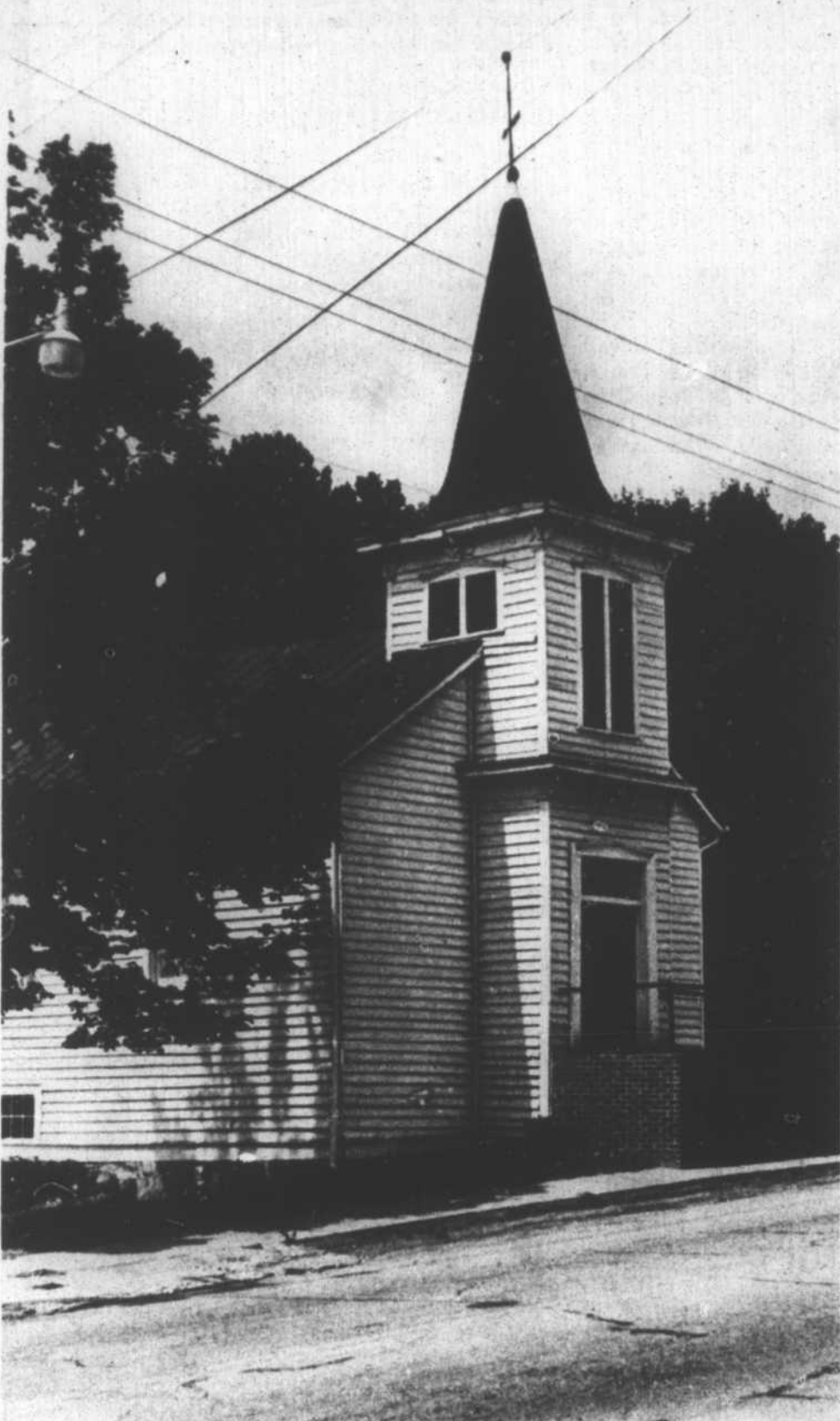
The U. S. Department of the Interior has approved a $3,000 grant to the N. C. Department of Cultural Resources for rehabilitation of the Oak Chapel AME Church on East Macon Street in Warrenton. The federal grant will be matched by $3,000 in local funds, Congressman L. H. Fountain announced. The program objective is to rehabilitate church steeple and replace deteriorated metal gutters and downspouts. Built prior to 1882, the church is a gable-end structure with an engaged tower, square in plan, with bracketed cornice at two levels with shingled tower. (Staff Photo)
