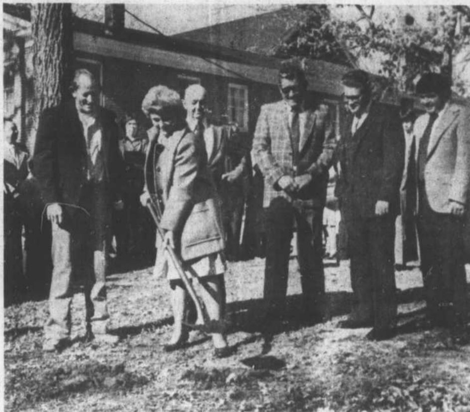
GROUNDBREAKING — Mrs. Lorene Mustian lifts the first shovel full of earth at the fellowship hall groundbreaking service recently at Sulphur Springs Baptist Church. Observing are Isadore Pitzing and Gordon Limer, committee members; Bob Kinton, chairman of Deacons; the Rev. Julian Mills, pastor, and Raeford Pernell, building committee member who will oversee the building project.
