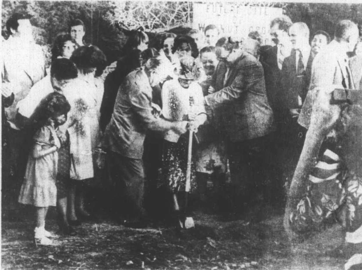
Groundbreaking ceremonies were held at the future site of the newly-formed Walnut Grove Baptist Church in Arcola on Sunday afternoon. Those shown participating in the digging of the first
