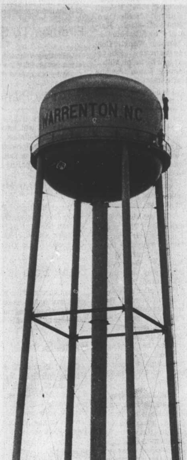
The finishing touches were put on the Warren County fire-radio system last week when these two Motorola representatives installed the repeater portion of the system on a communications tower adjacent to the Warrenton water tank. The system puts the 13 county volunteer fire departments and the Town of Littleton department on a countywide monitoring and alerting system. The installation of the repeater completed about three months of work at a total cost of about $98,000. (Staff Photo)
