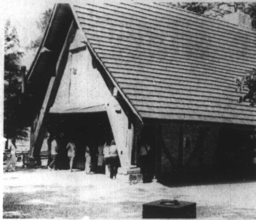
This large A-frame building contains the kilns used by glassmakers at Jamestown, Va. Craftsmen employed by the U. S. Department of the Interior turn out glass items similar to those produced nearly 400 years ago on the shores of the James River. Some of the tourists standing in line to purchase glassware are shown above. (Staff Photo)
