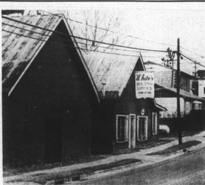
White's Building Supplies, Inc. on West Franklin Street, a 62-year-old Warrenton landmark, will this month close its doors and vacate the property which has housed the business since it was incorporated in January, 1923. (Staff Photo)
