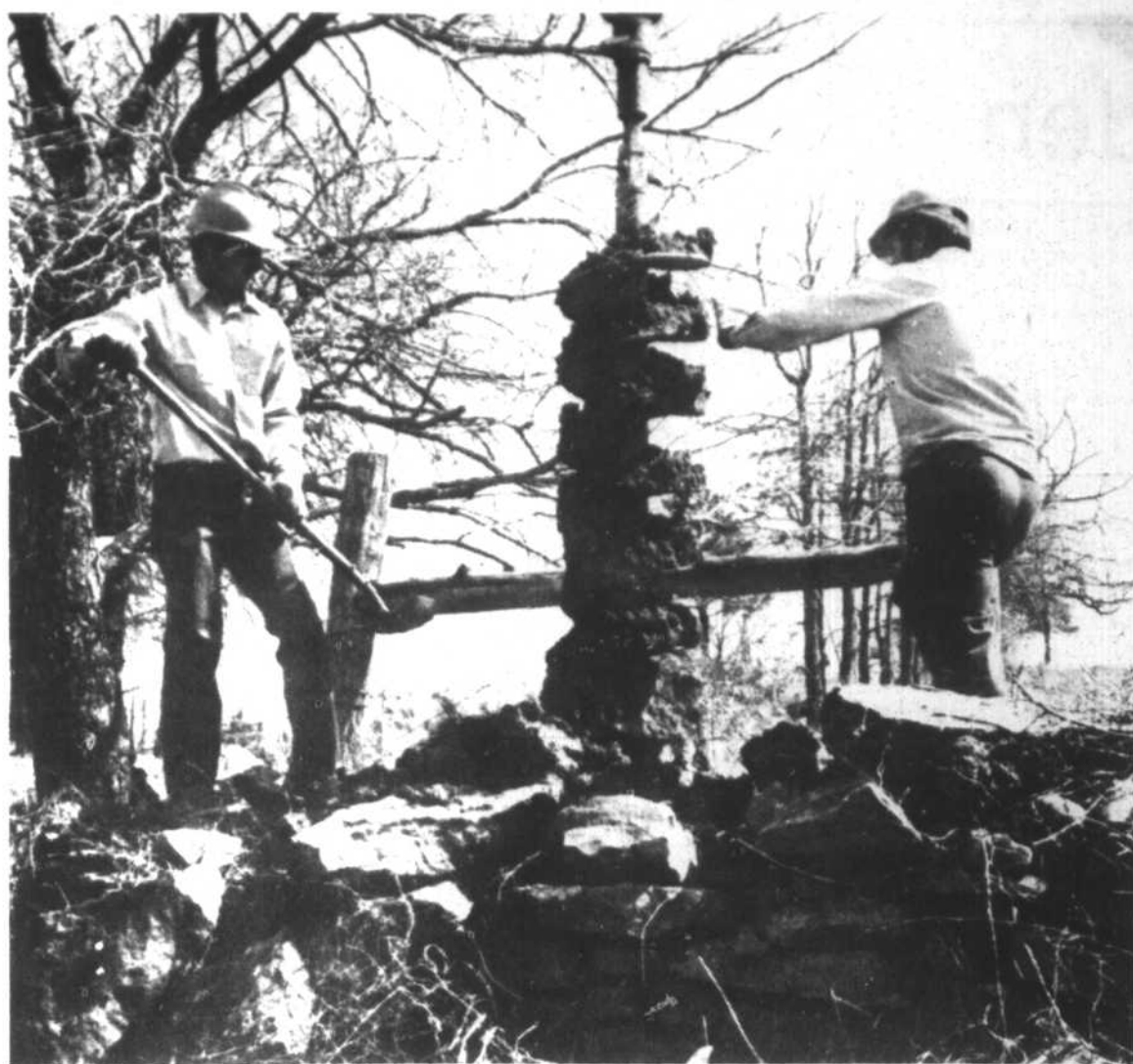
Mechanical auger bores into a northwestern Arkansas hillside as linemen prepare to install a new pole near Hogeeye. On such stonebound terrain, the Ozarks Electric Cooperative upgrades service for its 31,000 members along 4,810 miles of line.
