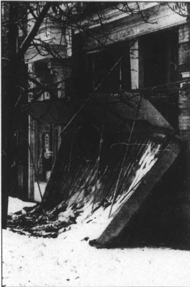
The icy coating which covered Warren County this week proved too much for this awning in front of Rennett's Beauty Supply on Main Street in Warrenton. It fell to the sidewalk Tuesday morning. (Staff Photo by Howard Jones)
