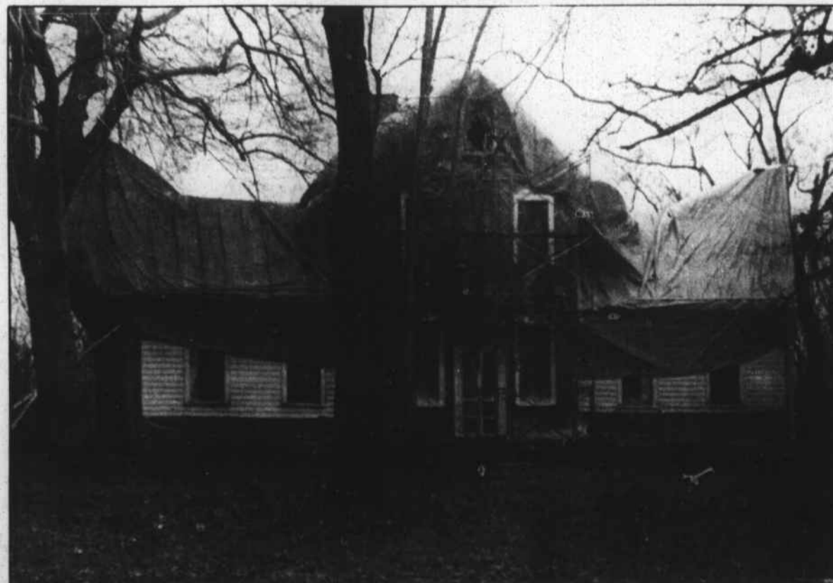
Looking every bit like an unwrapped package from the recent holidays, the historic Shady Oaks house south of Warrenton on Baltimore Road is covered with plastic to prevent damage by rain and
