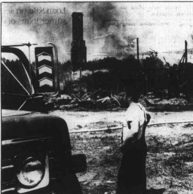
Ridgeway Fire Chief Reuben Holtzman surveys a house burned during a training exercise held last weekend. The structure was donated by Ben Hargrove. Other units participating in the exercise were the Soul City, Norlina and Drewry fire departments.
