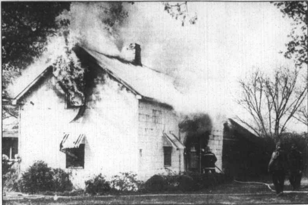
Firefighters are shown at the residence of Mrs. Lanie Hanes, located on the Oine Road, which caught fire last week due to a faulty wood stove that was located in the front room. The inside of the
