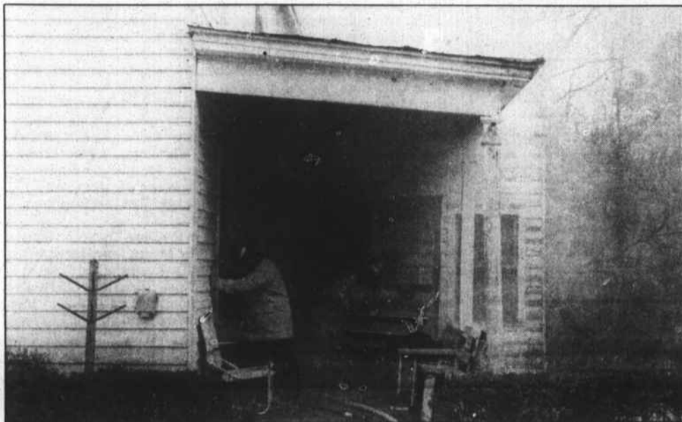
Firemen Work To Remove Smoke From Smoldering Residence
