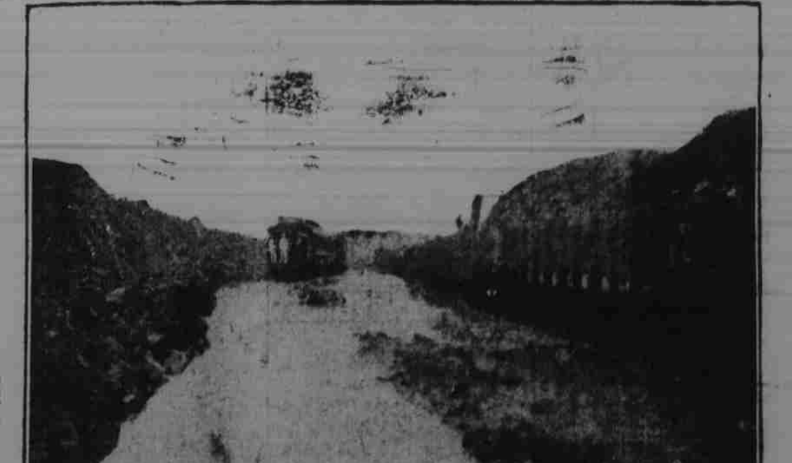
THE PRESIDENT'S TRAIN RUNNING THROUGH WATER IN THE CANAL DITCH. While President Roosevelt was inspecting the work done on the Panama canal his train ran along tracks covered by water in many places. The central figure on the rear platform of the last car is the president. At the right are cars loaded with rock and dirt.
