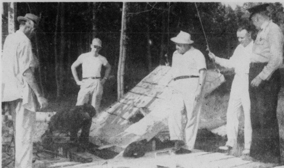
Lonnie Poole, Zebulon welder, is pictured filing the end of a joint of pipe in the deep well being drilled by the Heater Well Company for the Town of Zebulon. Each section of pipe had to be welded around the connector before being sunk. Poole's ground wire can be seen clamped to the pipe. Electrical connection for arc welding is made by touching the
