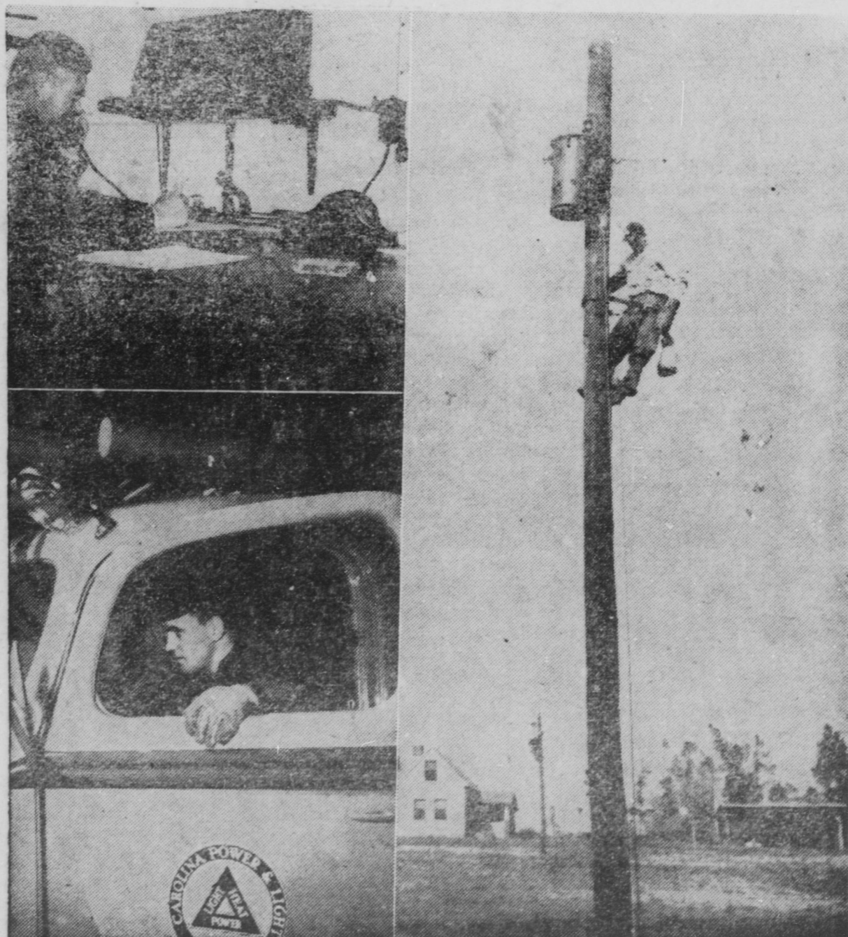
No more checking back into the office to pick up service complaints. Troubleshooters of Carolina Power & Light Company now are equipped with office-to-truck and truck-to-truck radios. Upper left, a divisional maintenance man calls a truck ten miles away. Below, a lineman gets the message. Right, the crew is on the job, putting juice in a remote farmhouse which in the old days might have been blacked out for a couple of days.
