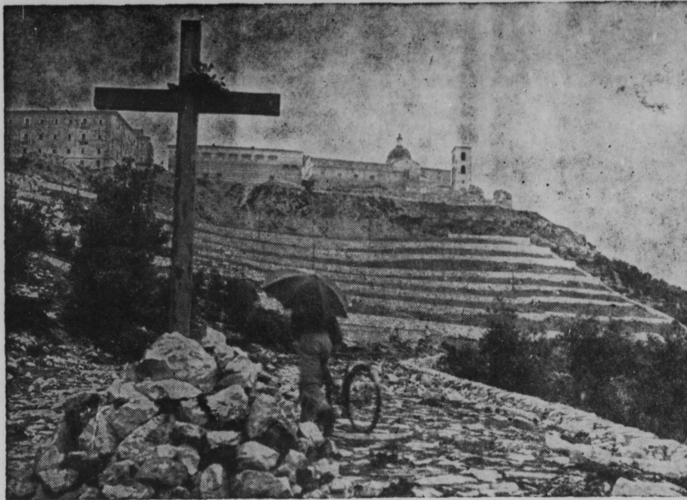
The historic Benedictine Abbey of Monte Cassino in Italy, victim of the saturation bombing in World War II when the Germans used it as a stronghold to hold up the Allied advance, is fast rebuilding. This recent photo shows the abbey with its walls rebuilt.
