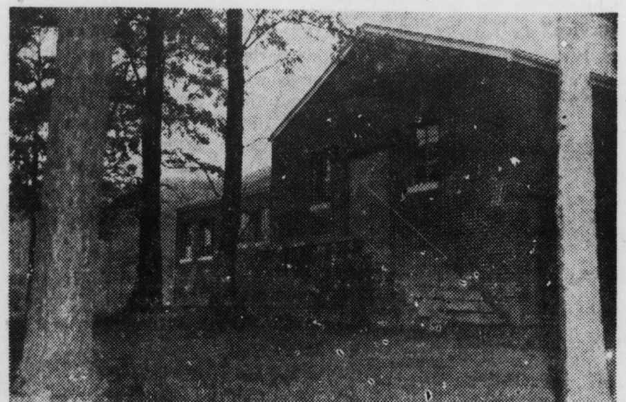
THE COMMUNITY BUILDING is important in a well-knit, friendly town. At Swannanoa, North Carolina, citizens realized the need, raised the money for materials, and built this one with volunteer labor. Every town needs a social and civic center.
