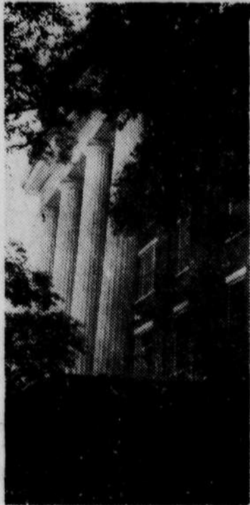
FRANKLIN ACADEMY BUILDING. Built in 1806, this building still stands, and is a historical landmark of Louisburg College.
