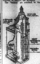
building by fasteners in holes drilled into the exterior terra cofta. Sprinklers are turned downward so they will drain, and are pointed directly at the windows. In case of danger from an outside fire, pumps are started, control valves on the top floor where the entire system is man-
