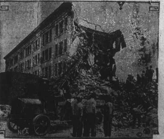
Santa Barbara is hard at work repairing the devastation wrought by her earthquake. This picture shows workmen busy on the ruins of the San Marcos building, which was one of the largest in the city.
