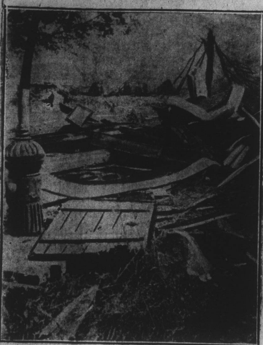
This hose, attached to a hydrant at the centre of the arsenal blast at Lake Denmark, N. J., was evidence that the explosion was started by a fire, caused by lightning, instead of the lightning ignited explosives direct. Marines were believed to have been fighting the fire when the blast came.
