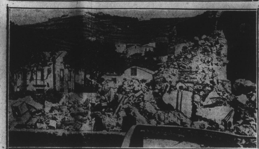
This is a general view of damage done when a series of earthquakes rocked Horta, in the Azores Islands. Many were killed.
