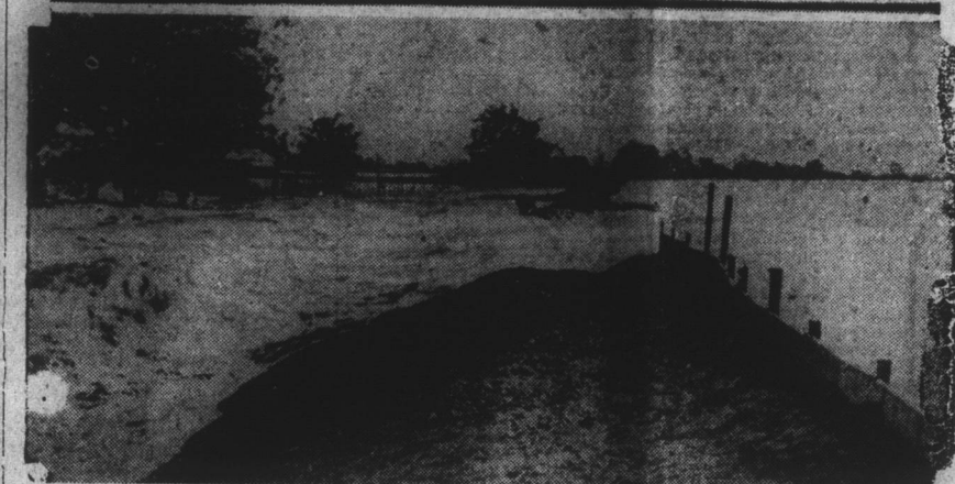
The Mississippi River is cutting a new channel to the sea through the Louisiana "sugar bowl." Picture shows one of the many breaks in the levee through which water, estimated at 500,000 cubic feet a second, is pouring.
