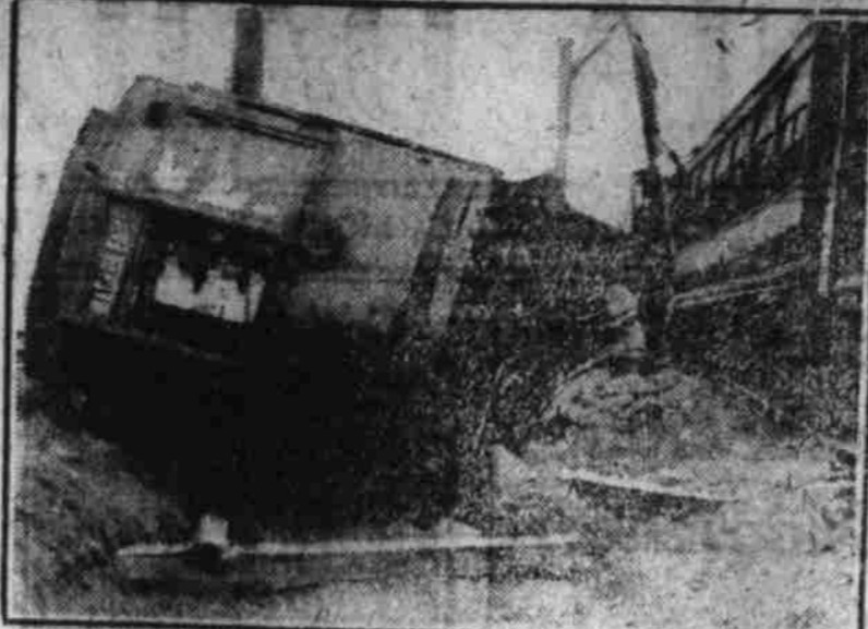
Several score persons were injured when a three-car electric train of the Niagara Falls "high speed" line was wrecked following a dynamite explosion near Buffalo, N. Y.
