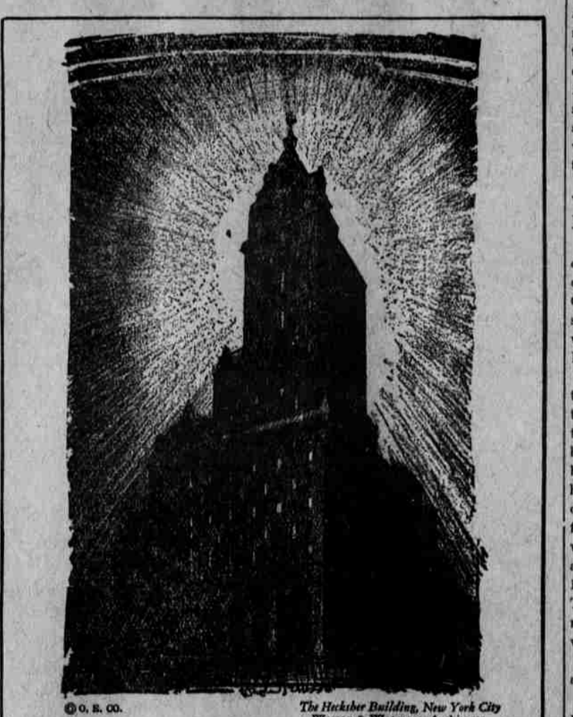
© O. S. CO. The Hecker Building, New York City Warren & Wetmore, Architects
