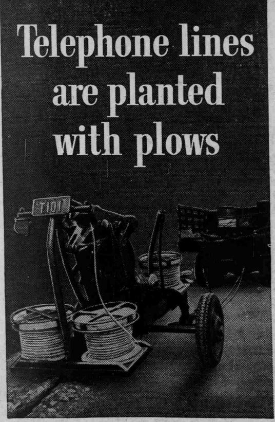
URAL telephone wire-not in cables-can now N go underground where bad weather and grass fires can't harm it.
