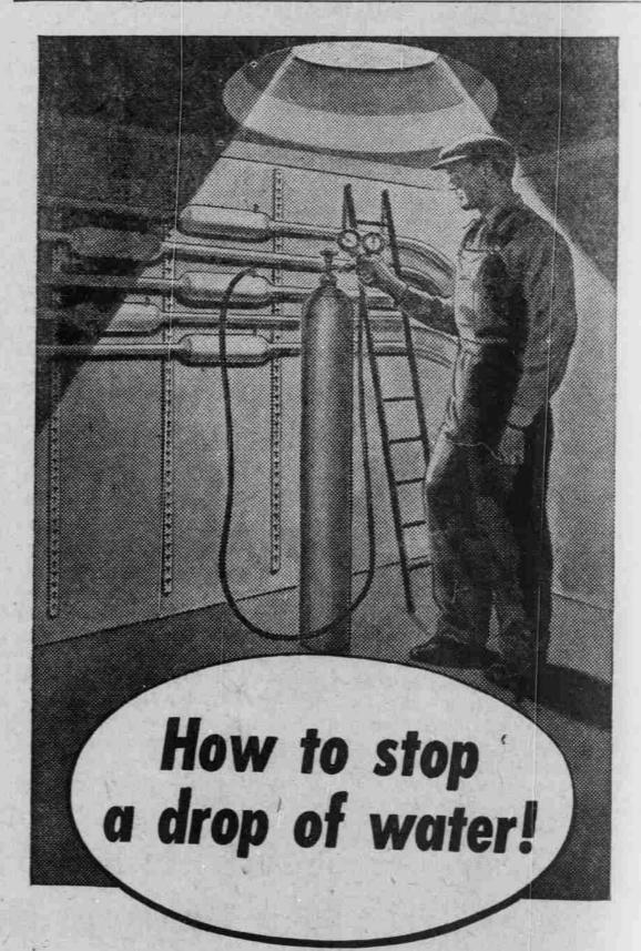
A tiny pin-hole in a telephone cable can admit moisture, causing short circuits and service interruptions. But Bell System men have found a way of beating this trouble to the punch.
