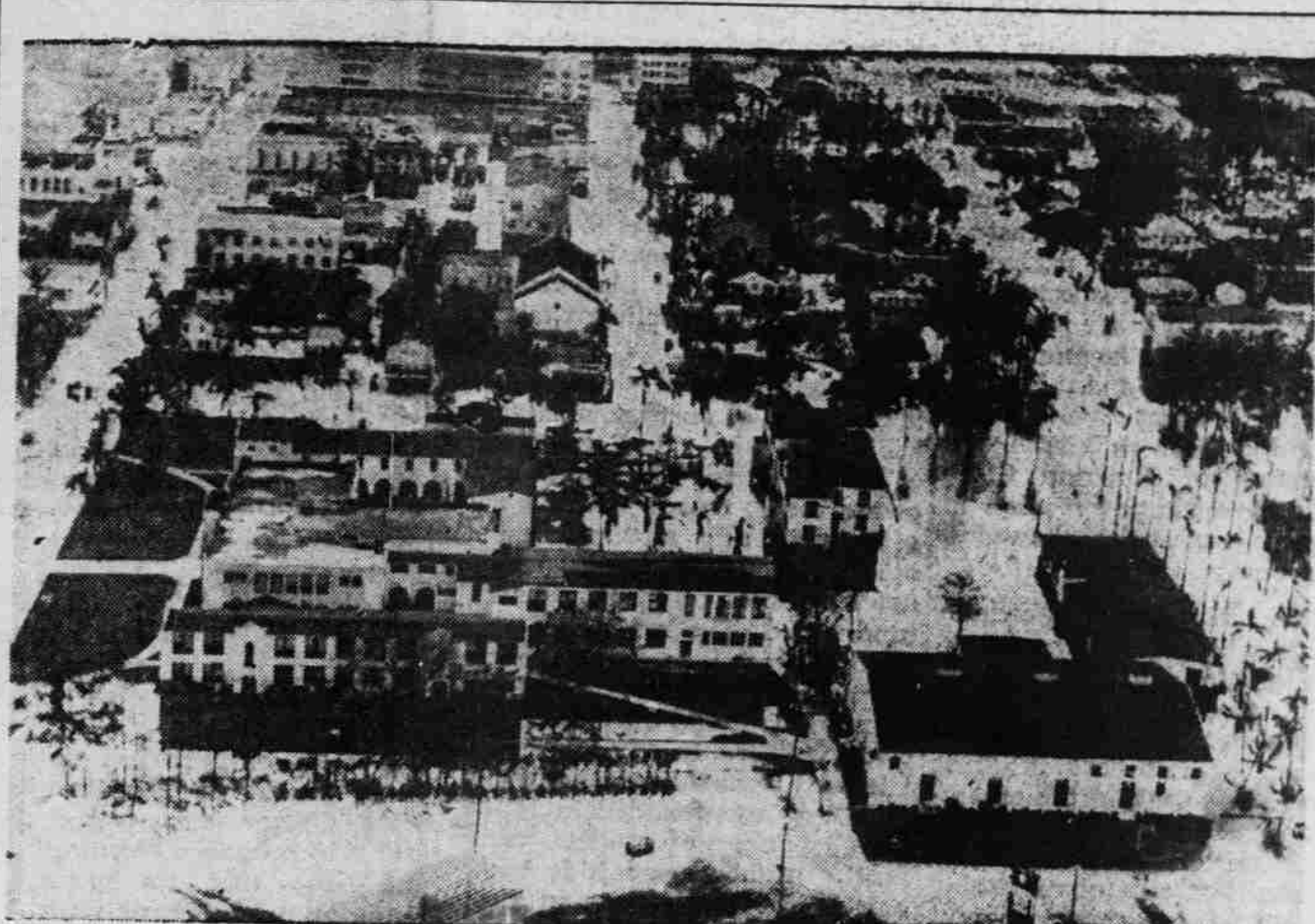
IN THE WAKE OF THE HURRICANE which swept across southern Florida, a final deluge of rain resulted in flood waters inundating a large area of Fort Lauderdale, above. The rising waters created grave problems of health and housing in many parts of the lower Florida east coast. The hurricane, which blew out to sea, turned back toward the coast states. (International Soundphoto)
