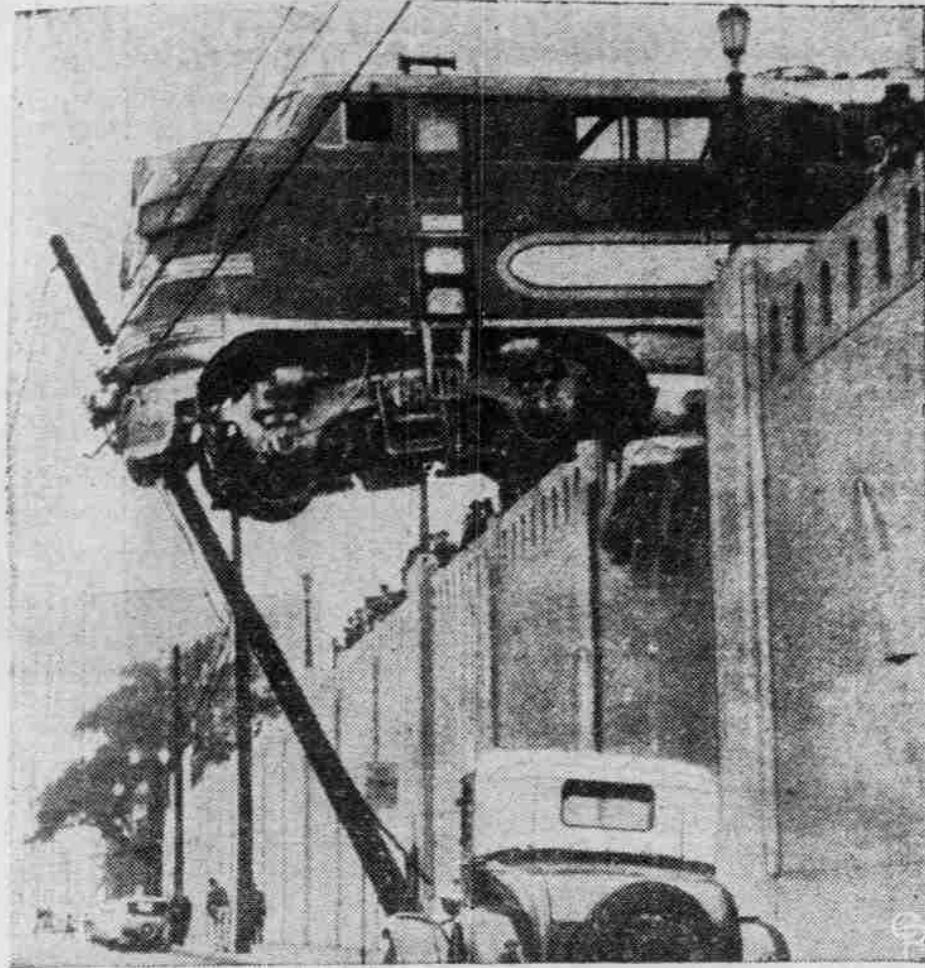
HANGING PRECARIOUSLY over a Los Angeles street is the locomotive of a four-unit Diesel engine train, which crashed through an 18-inch wall and came to rest against a power pole. The failure of the brakes to work was blamed for the freak accident, which occurred as the engine, after uncoupling its coaches, had started for roundhouse. (International)
