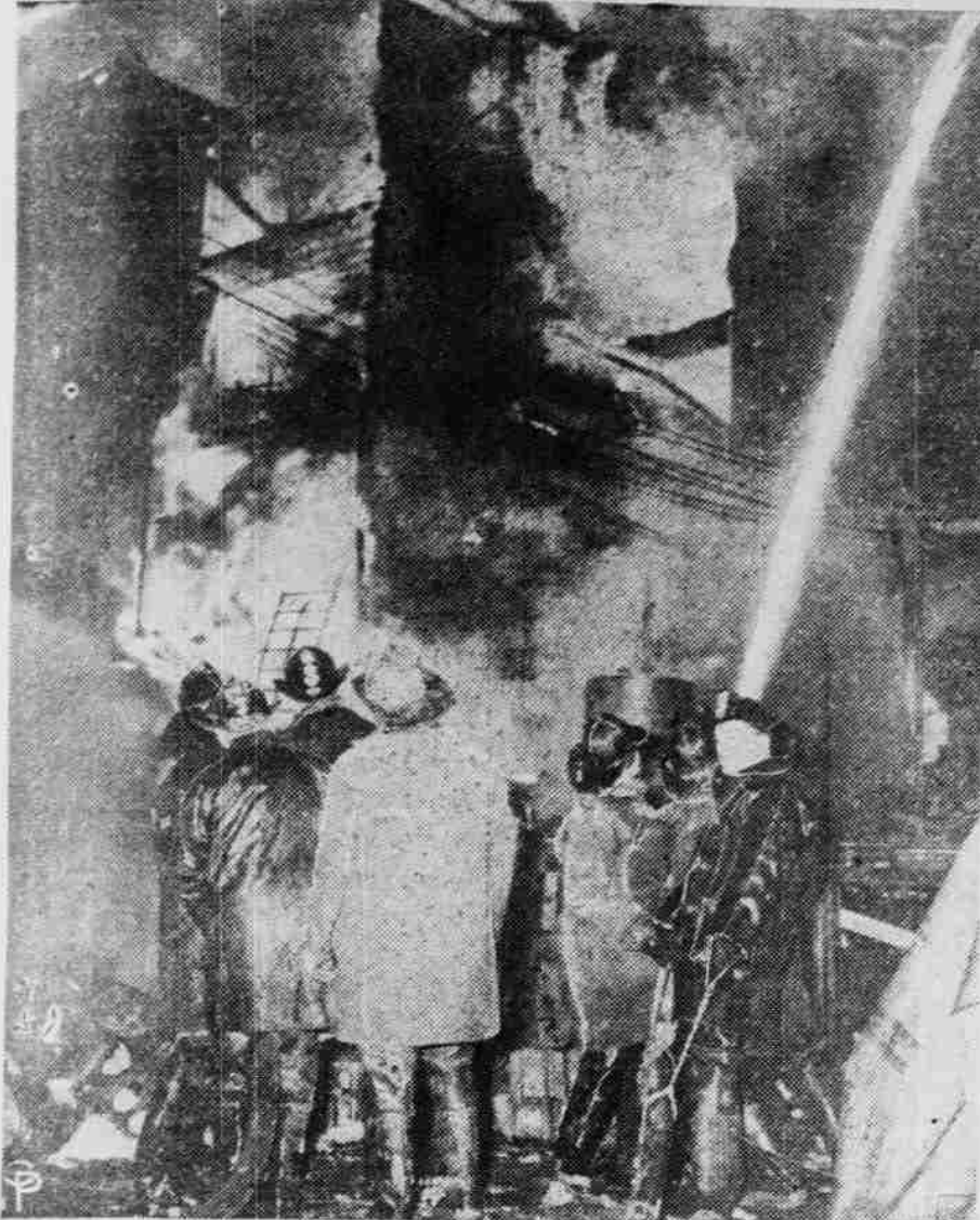
WHILE FLAMES ROAR THROUGH a furniture and carpet plant in Trenton, New Jersey, firemen shoot a stream of water onto an adjoining building in an effort to check the spread of the fire. Flames gutted four nearby buildings. Damage is estimated at about $1,000,000. (International)
