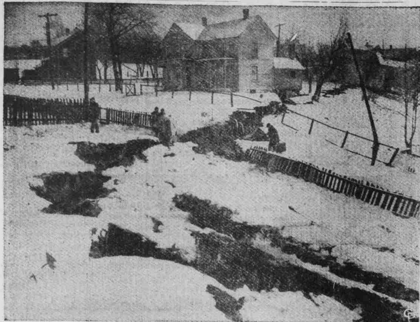
GAPING GROUND CRACKS in the anthracite mining town of Carbondale, Pa., caused by a mine cave-in give the appearance of an earthquake's visit. Houses buckled and tilted on their foundations, breaking water pipes and flooding basements. Four persons were injured.
