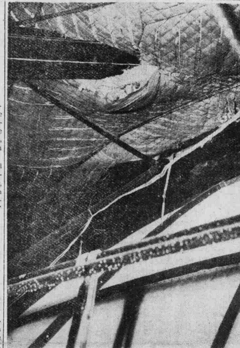
A FIRE ABOVE THE DOME in the Morehead planetarium chamber Tuesday morning damaged acoustic materials which had not been fireproofed. A portion of the material burned is shown suspended above the back surface of the dome. Officials reported that the $115,000 stainless steel dome was not damaged. The part of the dome shown in the lower right part of the picture suffered only water damage. Flames were ignited by sparks from a worker's blowtorch which caught in a pocket of the material. Purpose of the material is to remove all reverberations and echo during a demonstration in the planetarium chamber below.
