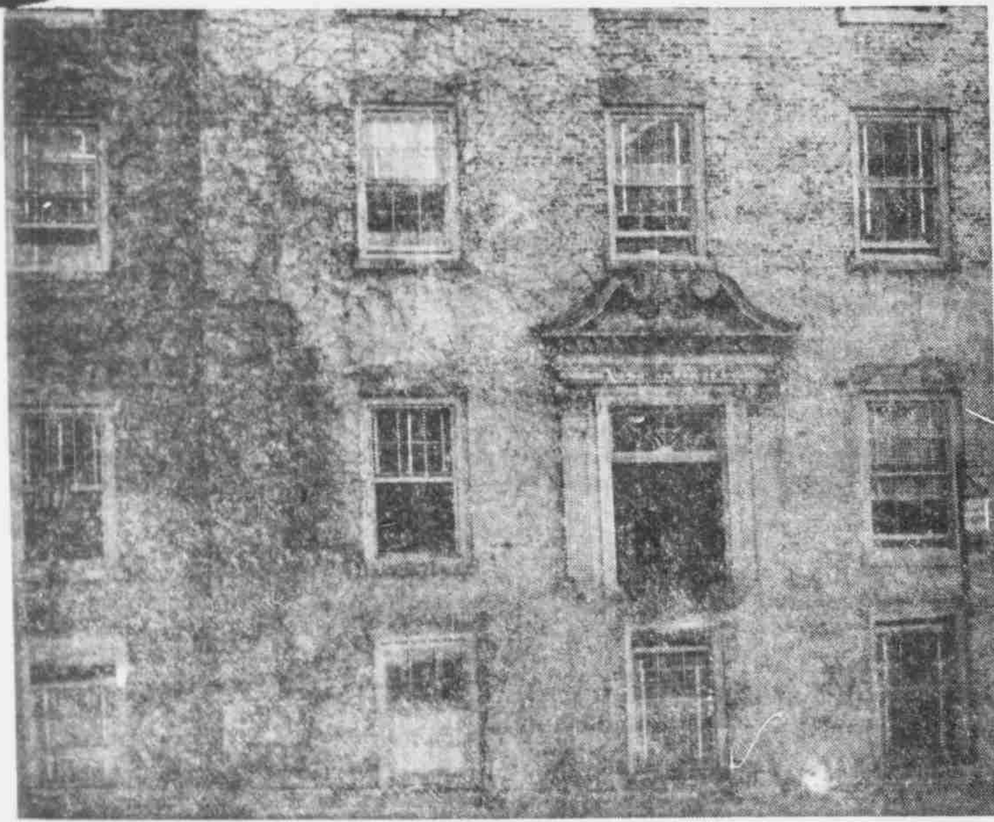
SOGGY but standing, South Building, rises above the receding flood waters, a saturated symbol of strength. Photo by Ron Cunningham
