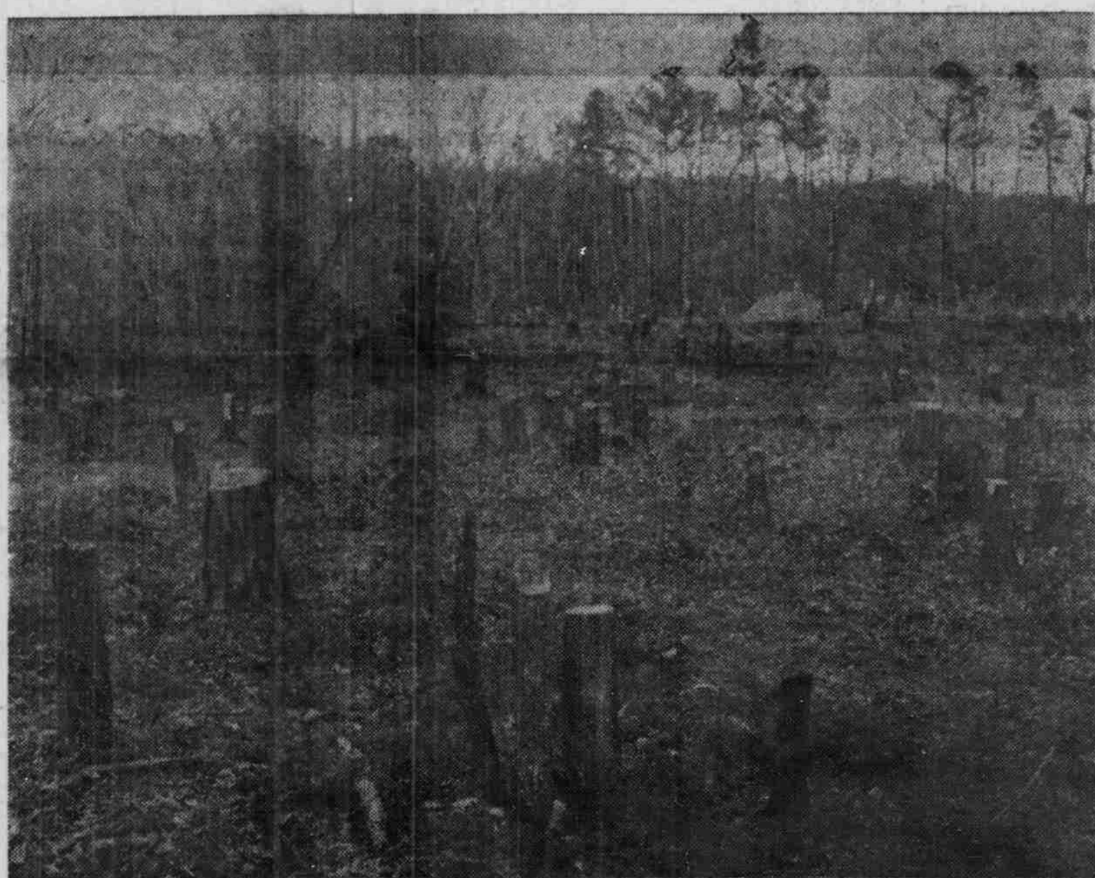
NEW DORMS SITE—Several acres of land is in the first stages of being cleared as the site of two new Carolina men's dormitories. To be built at a cost of $3,633,000.
