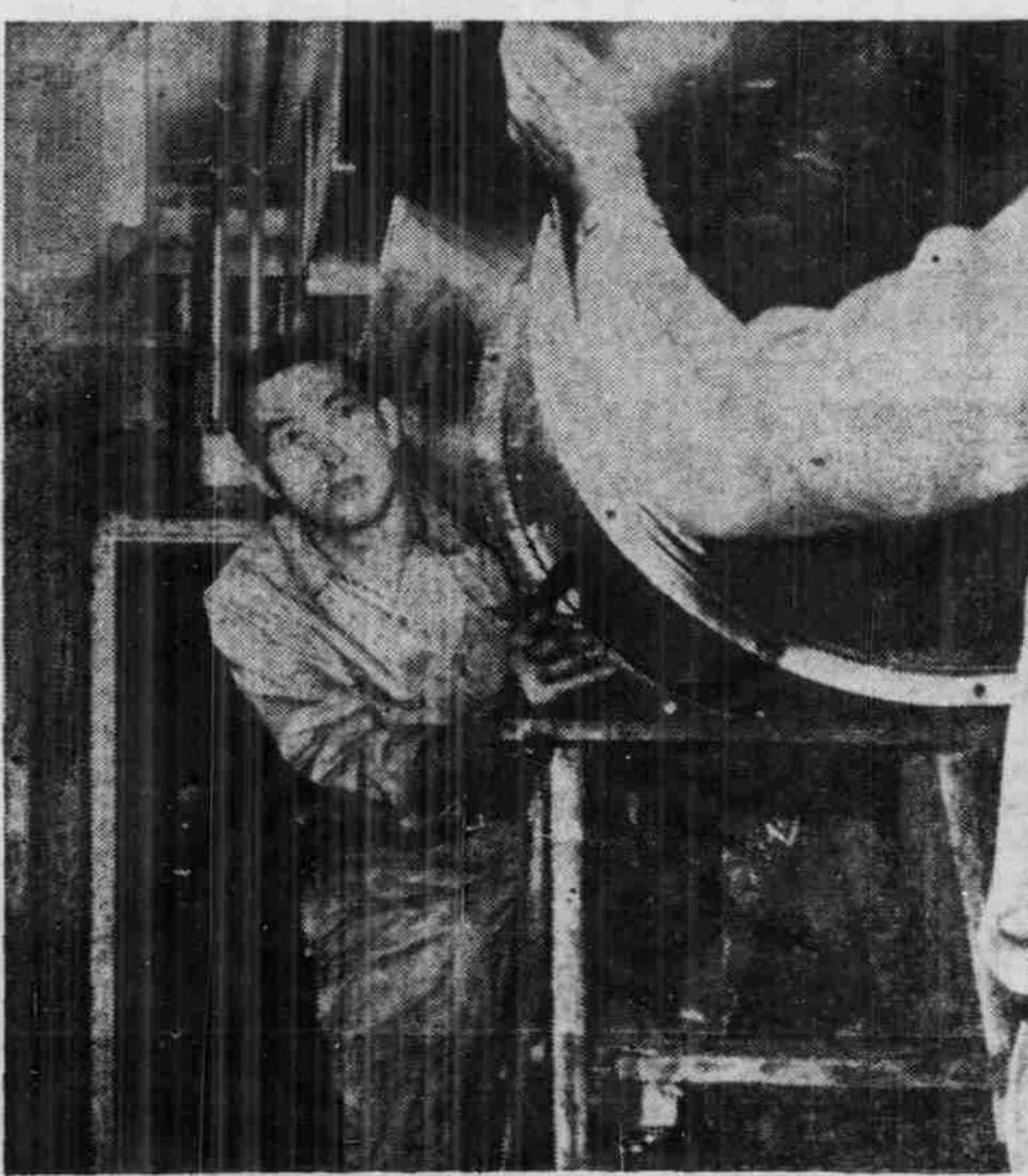
REMODELING: Two workmen install a ventilation unit in the Pine Room, now in the process of being remodeled. The Pine Room is scheduled to reopen November 15 with improved kitchen facilities, a new snack bar and cafeteria.
