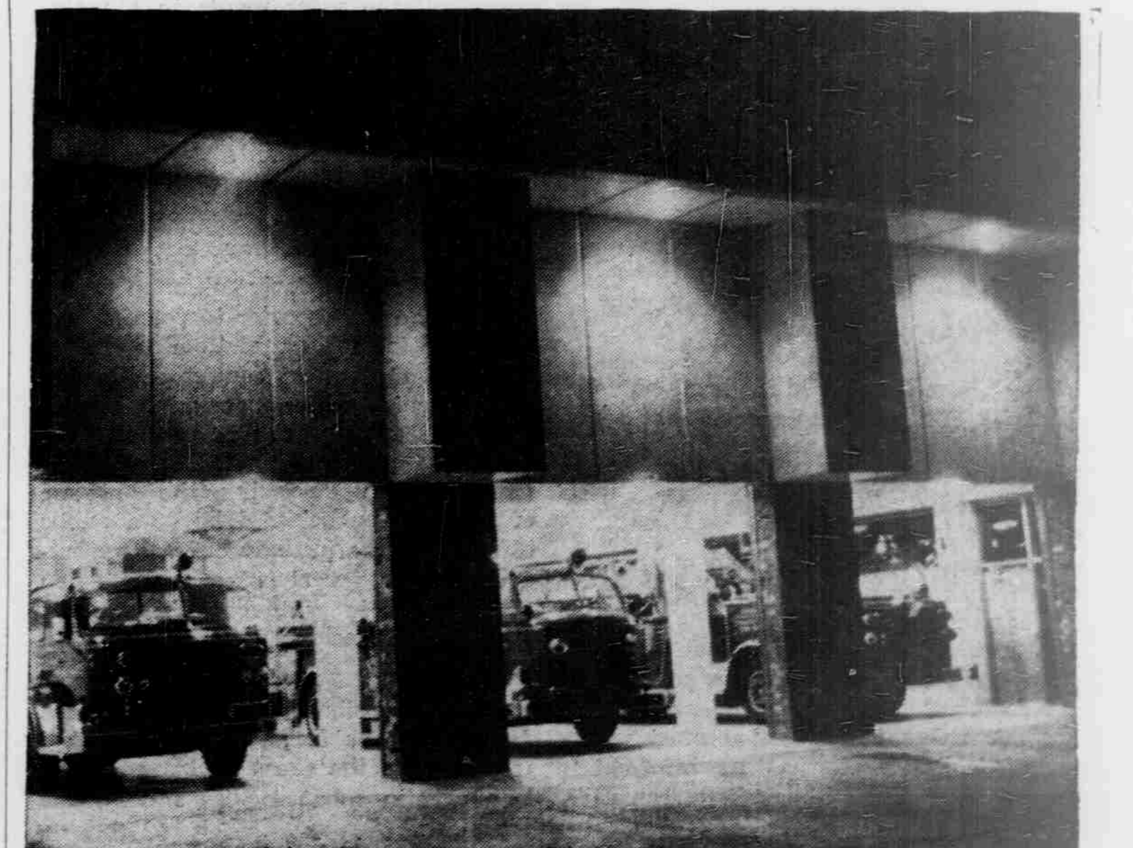
THE LIGHTS burn brightly far into the night at the new Chapel Hill Fire Department. The new building, an ultra-modern affair, provides the firemen with far more room than their old cramped quarters in the Town Hall. The new building is staffed by at least four men 24 hours a day.
