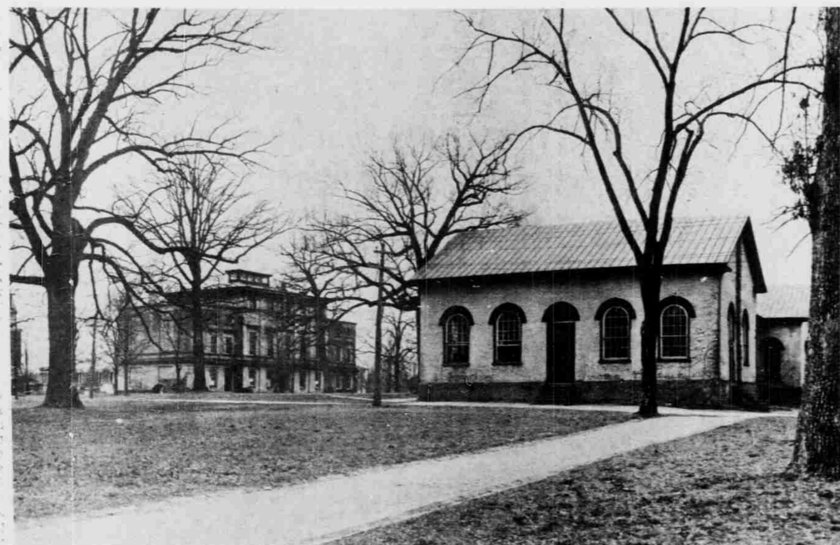
PERSON HALL IN 1919, showing wash and paint. Built as a chapel. Person was given arched windows instead of rectangular windows as on other campus buildings.
