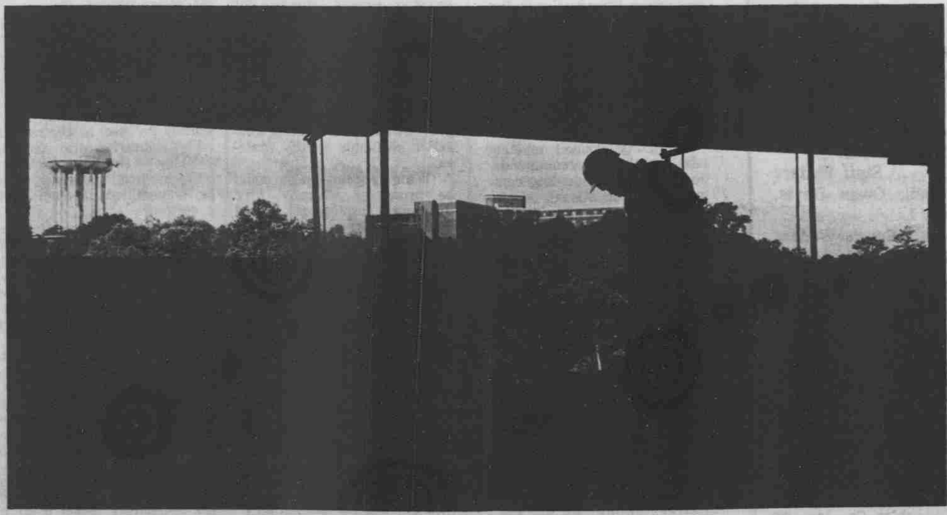
Workmen Brick 6th Floor With Morrison In Background
