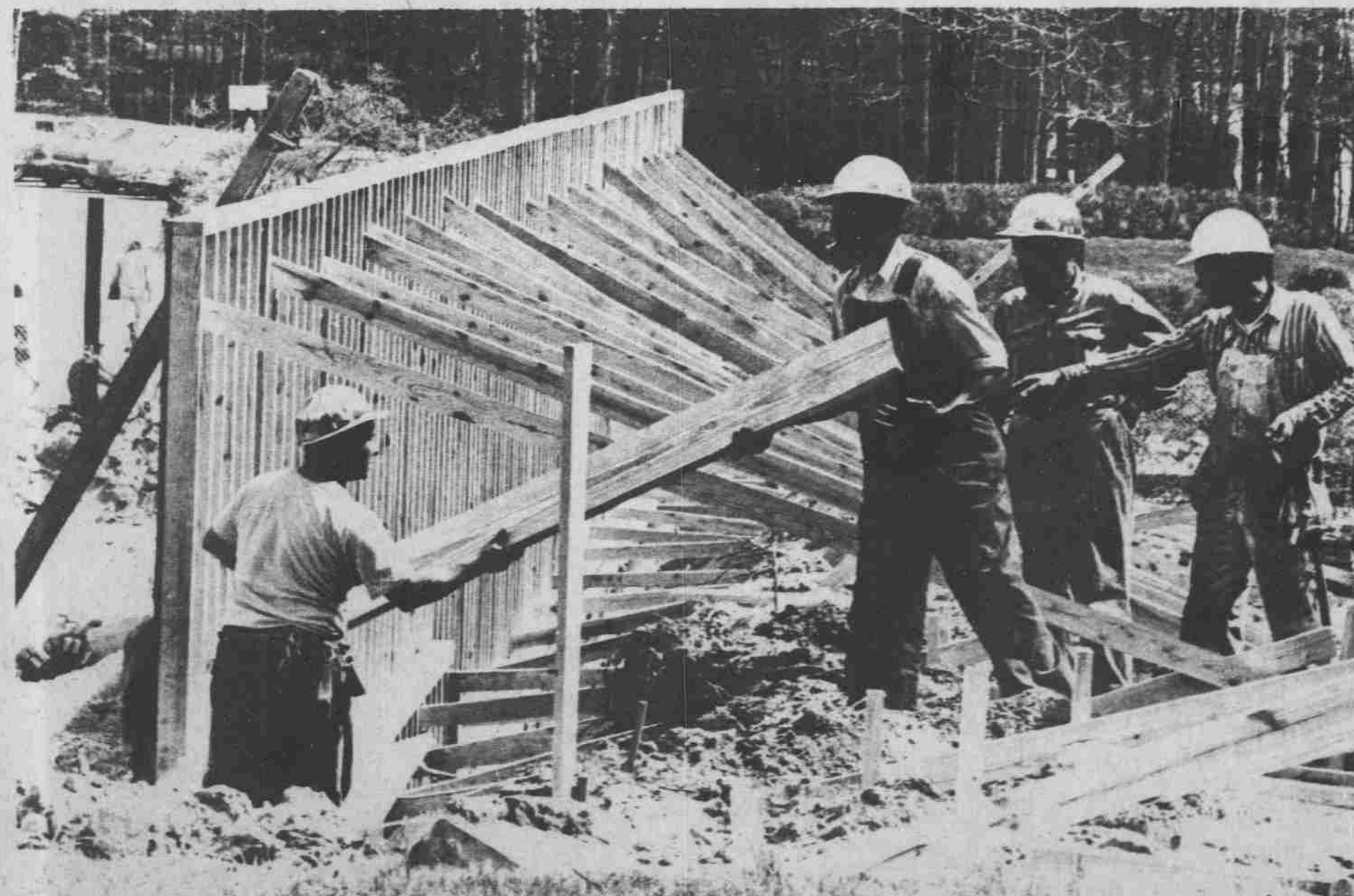
WORKERS BEGIN on the forms for the foundations of the new undergraduate library, which occupies part of what was the Wilson Library parking lot. Contractors say that the building is ahead of schedule and should be ready by June, 1968. —DTH Photo by Steve Adams
